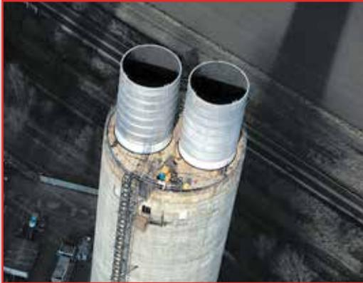
The global power generation industry relies on our unique **PENNGUARD™ Block Lining System** for long-term corrosion protection in their stacks. This versatile lining system is even suitable for seismic zones and can be applied over steel, concrete, gunite, brick, and fiberglass structures.
