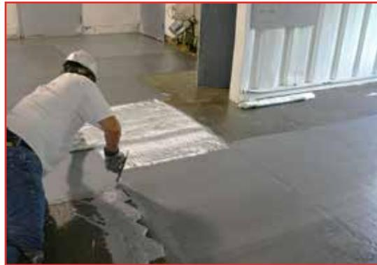
Compared with trowellable **PENNTROWEL™ Surfacer Systems**, **PENNTROWEL™ SB Systems** are applied using less labor-intensive slurry-broadcast installation techniques. These methods yield a non-slip, durable broadcast floor finish.
