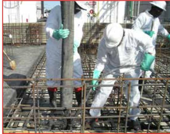
**TUFCHEM™ Silicate Concrete** is an acid-resistant substitute for Portland cement concrete. This active pharmaceutical ingredient plant, which uses strong sulfuric and acetic acids, constructed secondary containment dikes using **TUFCHEM™ Silicate Concrete** that was mixed on site in a continuous volumetric mix truck.
