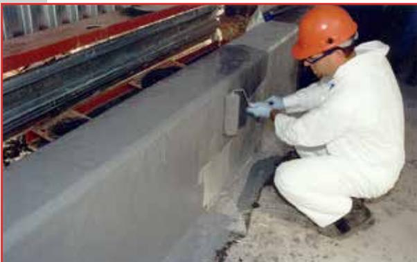
Flake fillers in our **PENNCOAT™ Lining** formulations reduce the lining's permeability for longer life in immersion service. Systems are designed for brush, roller, trowel, and spray application.
